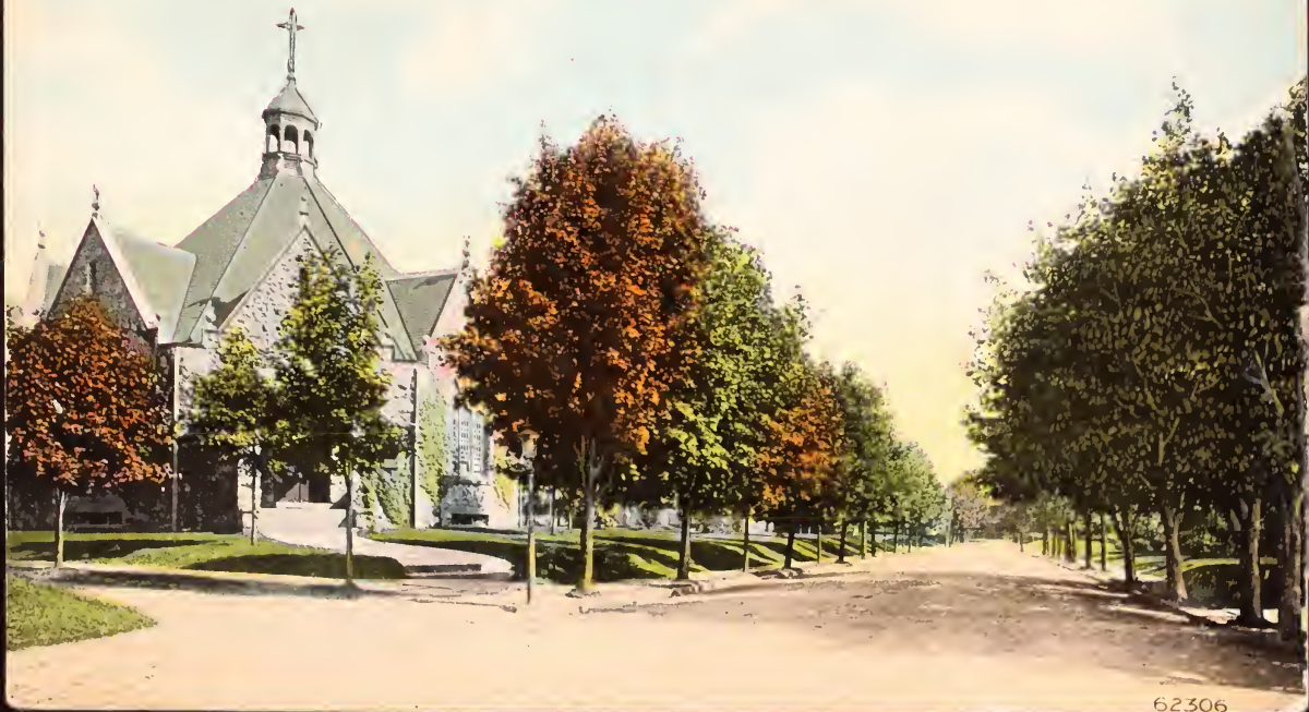
Monroe Street showing Presbyterian Church, College Hill, Easton, Pa.
